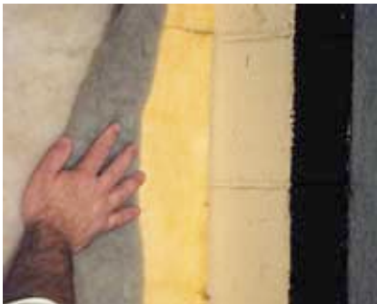
The insulation of the walls in both studios.
